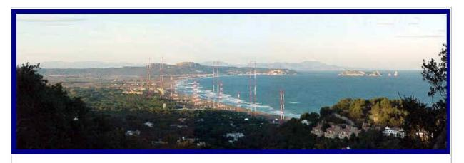
These four units, when combined as a million-watt transmitter, could be tied into the largest short-wave antenna in the U.S. inventory, a gigantic, ultra high-gain 4 x 8-stack array, arranged on eight towers, four of which are over 500-feet high with antenna curtain widths reaching nearly the length of a football field. A truly imposing sight as seen on beautiful beach property on the Balearic Sea roughly 60 miles north of Barcelona.
